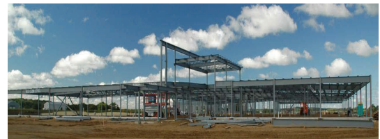
Construction of the new Osceola Medical Center Building
